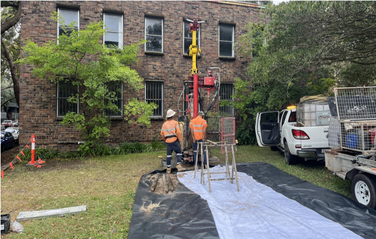
Figure 2-Photo of the drilling setup.
